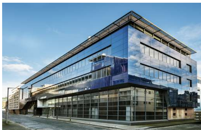
Fleming Court, Fleming's Place - Dublin (Irlande)
